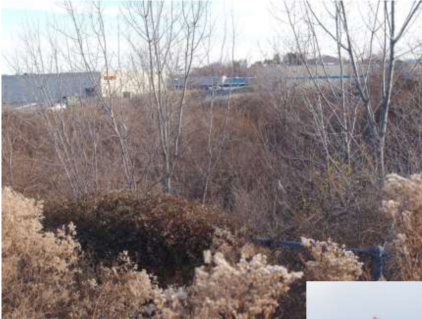
This fenced in retention pond near Ollies store in West Mifflin was overgrown with small trees and unmanaged weeds and invasives.
